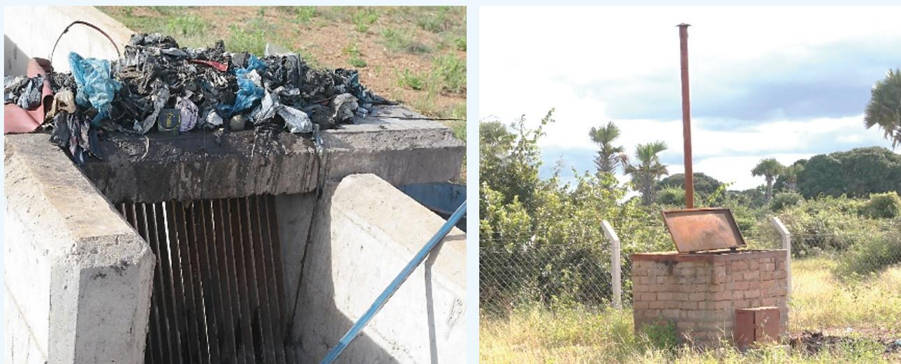
**Figure 4- 8 : Solid waste collected at bar screen (left) and a typical incinerator (burning chamber) (right)-Kahama**
