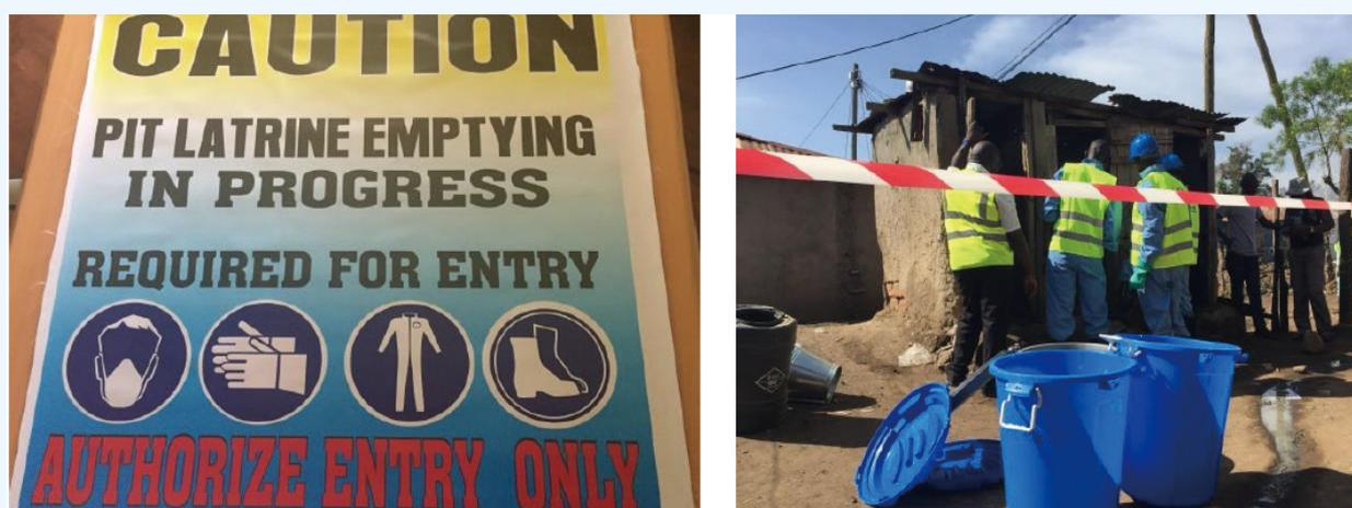
*Figure 4- 6: Sample hazardous workspace signage (Left), Barrier tape erected around workspace (right).*
